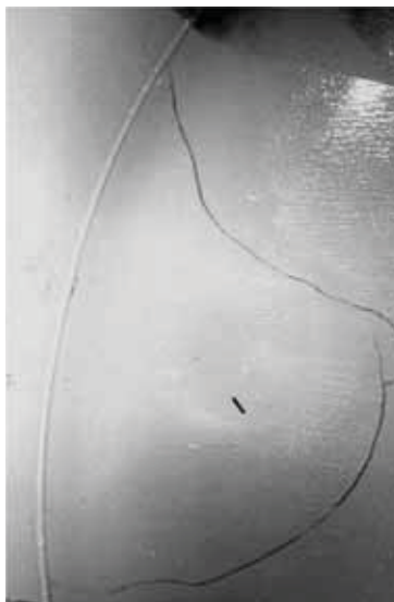
Figure 18.2 Cracks in the Inner Tank Shell
